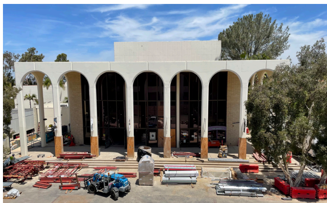
The Don Powell Theater renovation project at San Diego State.
