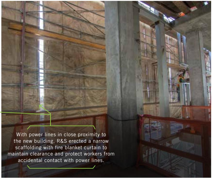
With power lines in close proximity to the new building, R&S erected a narrow scaffolding with fire blanket curtain to maintain clearance and protect workers from accidental contact with power lines.
