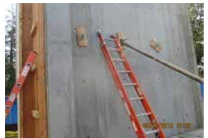
Further quality measures entailed construction of a two-story mock-up of several exterior building conditions. All team members heavily scrutinized and carefully inspected the mock-up, learning and resolving many challenges before beginning work in the field. This massive preplanning effort significantly contributed to achieving a high degree of aesthetic and waterproofing quality for the exterior skin.
