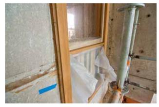
△ In addition to repairs and restoration of the different combinations of sliding windows, solid panels, louvers, the 203 teak window walls are also receiving much needed waterproofing.
